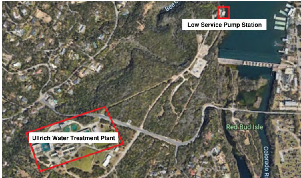
Figure 2.6.2: Ullrich WTP and LSPS Facilities Plan, Not to Scale (Image from Google Earth)
