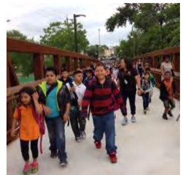
The North Acres Bridge provides a safe route for children to get to Hart Elementary. It was funded by the City of Austin and a federal grant.
