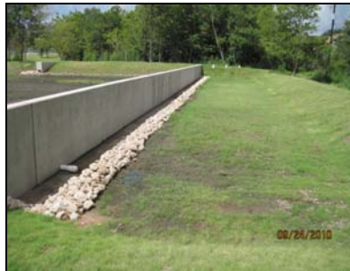
Warehouse Row Biofiltration Pond
