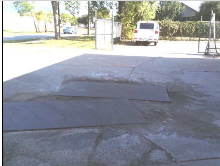
Driveway at Fire Station 24, 5811 Nuckols Crossing
