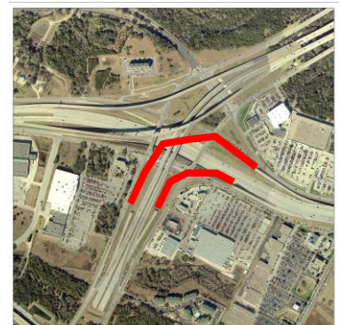
US 290 at Loop 1 Interchange Completion
