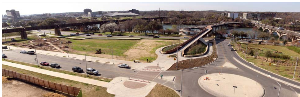
Pfluger Bridge Extension, part of Sand Beach Improvements
