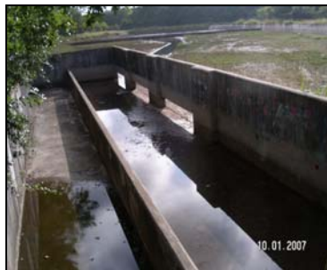
Brodie Lane Biofiltration Pond
