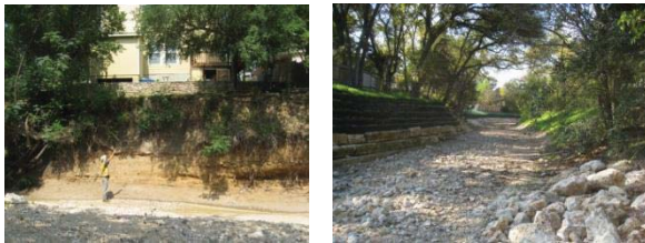
Fort Branch Eleanor Street Channel Rehabilitation (before and after)
