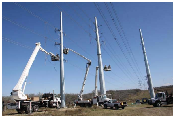
Installation of transmission poles at the Dunlap substation
