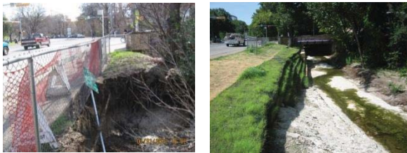
Waller Creek at Dean Keeton Bank Stabilization (before and after)
