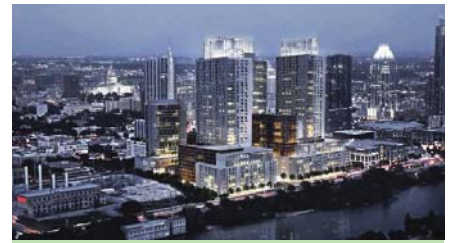
Green Water Treatment Plant and Seaholm District Redevelopment | p. 100
