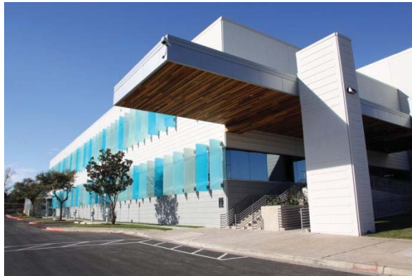
Completed System Control Center
