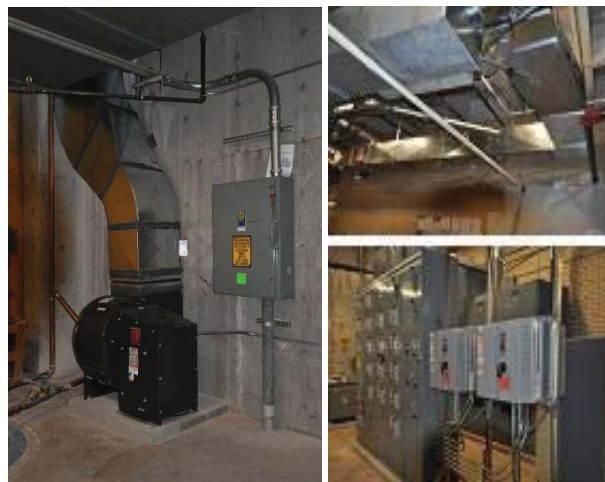
Faulk Central Library/ Austin History Center Chiller/ Cooling Tower Retrofit
