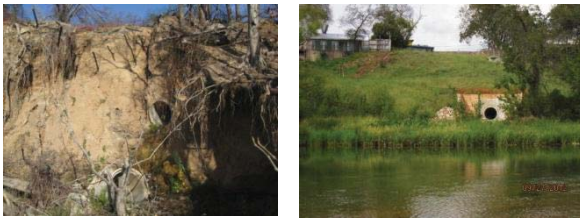
Colorado River at Tillery Street Stormdrain Outfall Stabilization (before and after)
