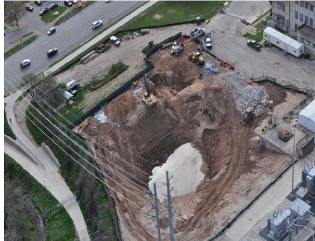
New Central Library Construction Site
