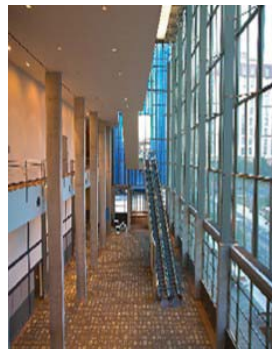
Escalator replacement and repairs at the Convention Center | p. 186
