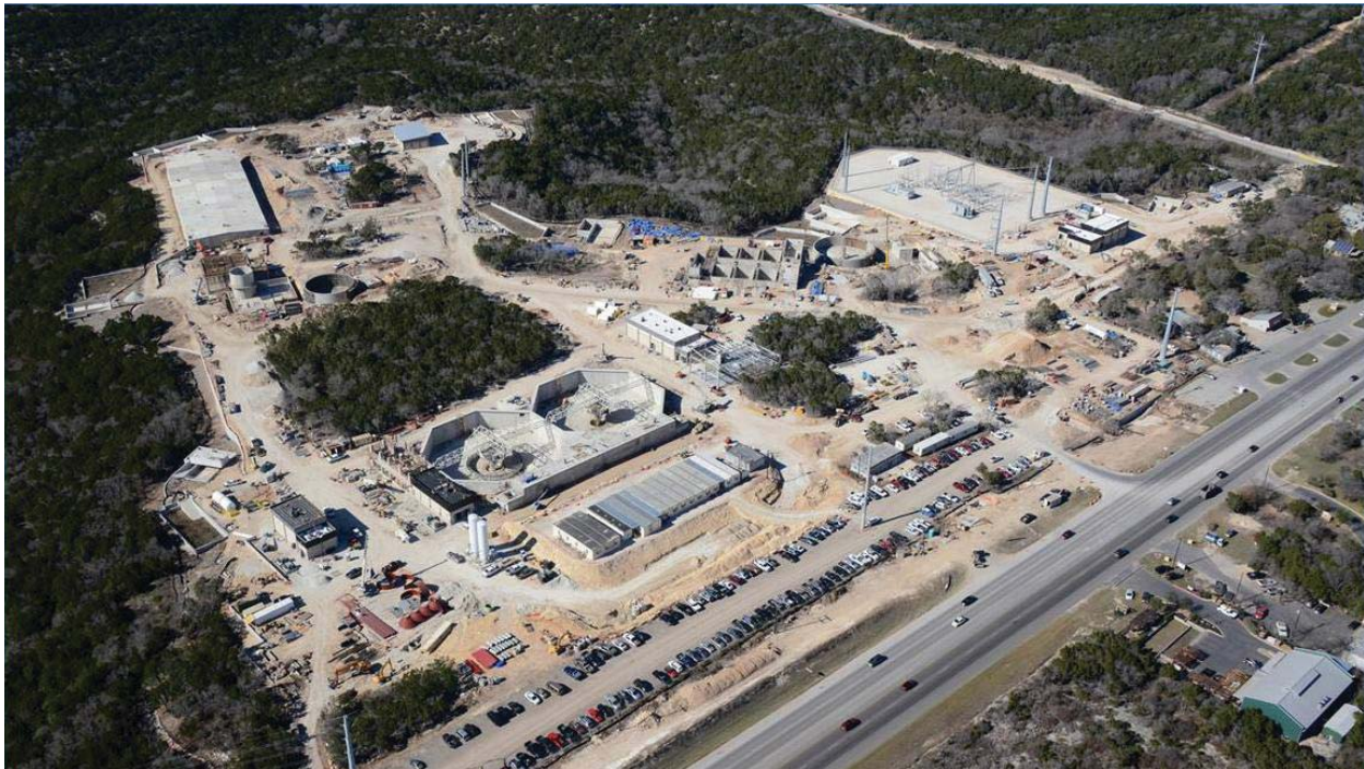
Water Treatment Plant 4 Site at Bullick Hollow
