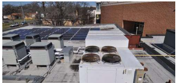
Carver Branch Roof
