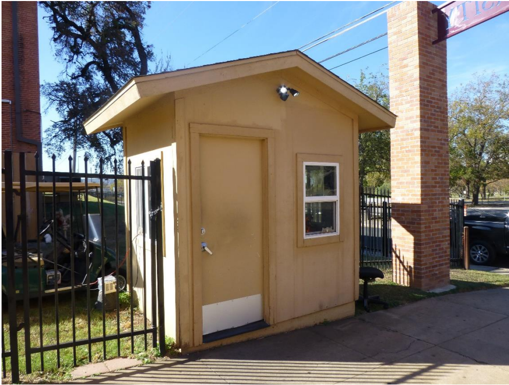
Photo 23: West Security Station, Huston-Tillotson University, looking southwest. 11/17/2020.
