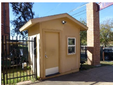
Resource 17 Name: West Security Station Resource Type: Building Stylistic Influence: None Year Built: Unknown Status: Noncontributing Photo(s): 23
