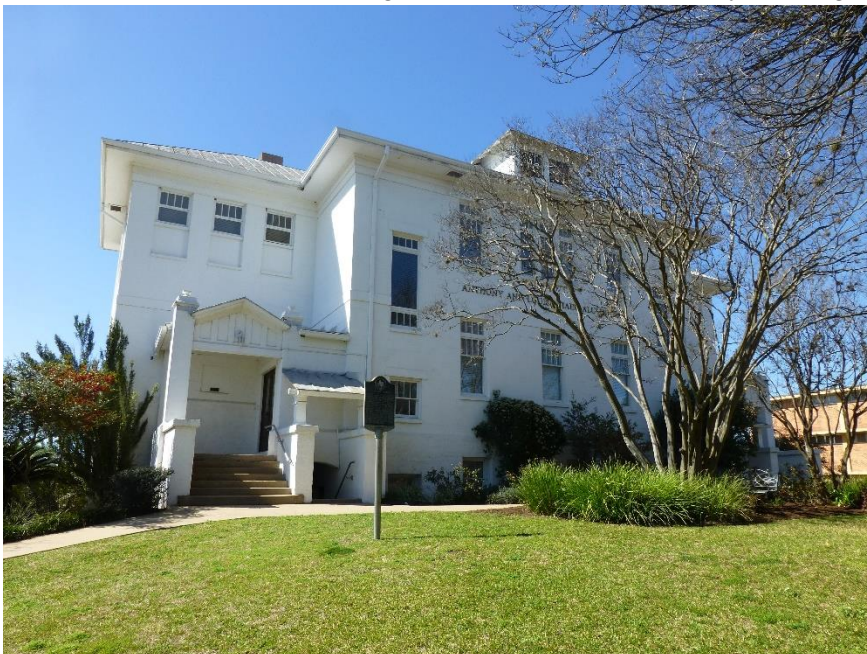
Photo 2: Administration Building, Huston-Tillotson University, looking southeast. 3/13/2019.
