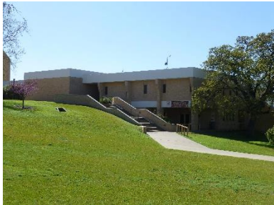
Resource 11 Name: Jackson-Moody Humanities Building Resource Type: Building Stylistic Influence: Brutalist, New Formalist Year Built: 1974 Status: Contributing Photo(s): 14-15
