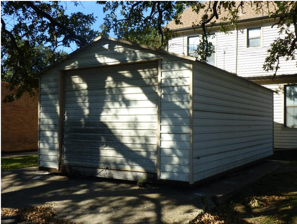
Photo 26: Storage Building (east), Huston-Tillotson University, looking west. 11/17/2020.
