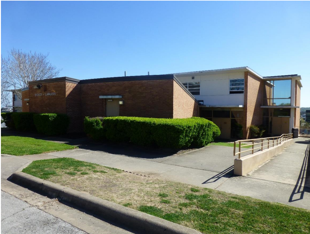
Photo 6: Dickey-Lawless Science Building, Huston-Tillotson University, looking southeast. 3/13/2019.
