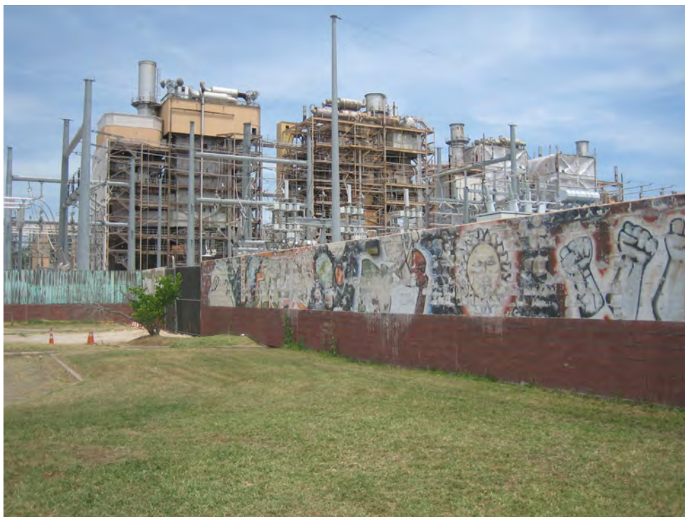
The Holly Street Power Plant was decommissioned in 2007. Since then, the surrounding neighborhood has seen reinvestment.
