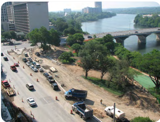
Construction of the Great Streets enhancements to Cesar Chavez.
