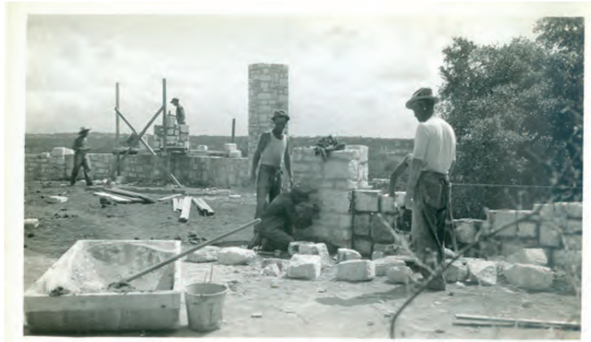
Lookout Point construction, 1934, Austin History Center
