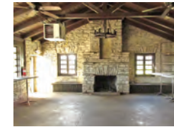
View to the south of the Main Room. An interior photograph from the 1940s shows a door opening in the southwest corner, now infilled.
