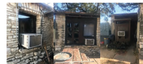
Figure 3: Caretaker Window Units
