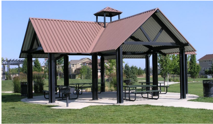
A. Covered Pavilion
