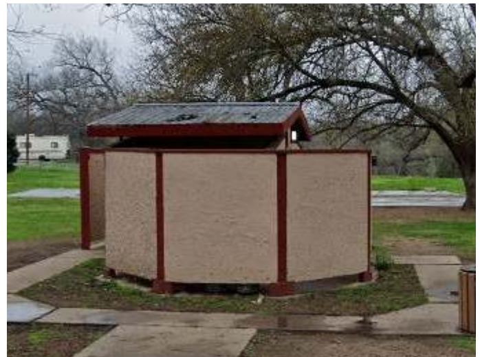
Zilker Restroom on the South Side of Barton Springs Pool
