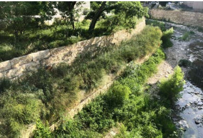
Limestone terraces along Waller Creek to slow down water flow
