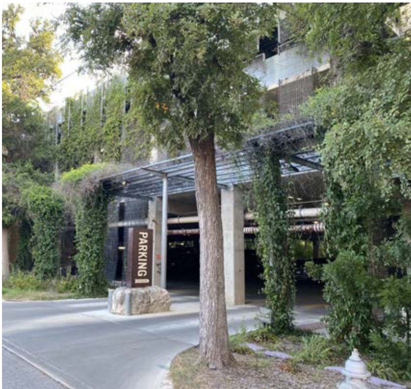
Parking Garage at Brackenridge Park
