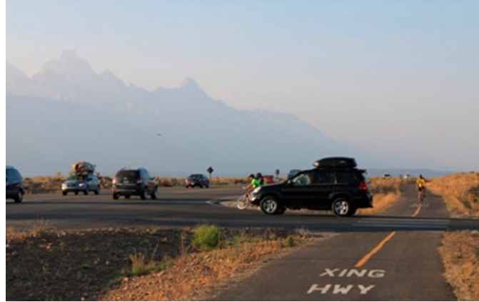
A SHARED USE PATH ALONG THE UNDIVIDED HIGHWAY 89 IN GRAND TETON PARK (PHOTO COURTESY OF U.S. DOT).
