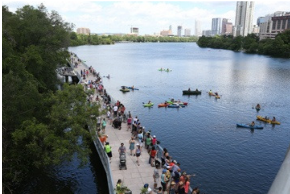
THE BOARDWALK TRAIL COMPLETED IN 2014 AND PICTURED ON OPENING DAY, COMPLETES THE BUTLER TRAIL LOOP AND PROVIDES BICYCLE ACCESS TO EAST RIVERSIDE AREA.
