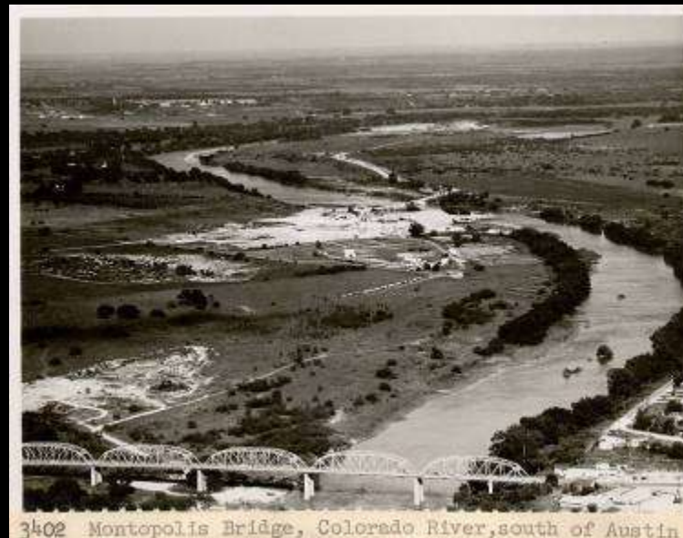
3402 Montopolis Bridge, Colorado River, south of Austin
