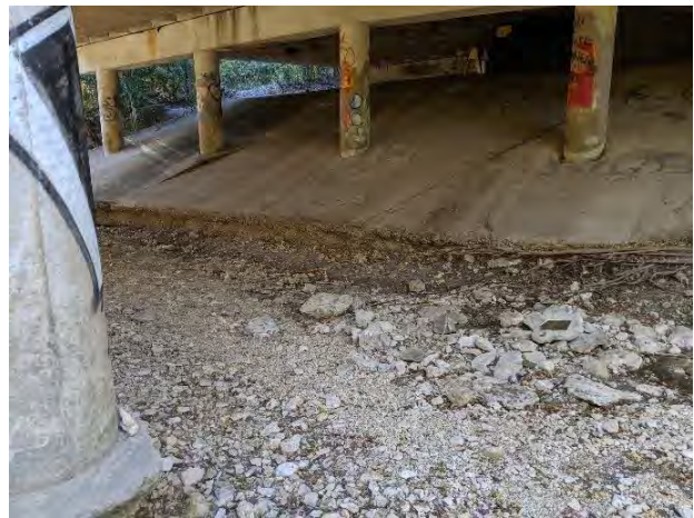
Figure 2-2. Williamson Creek at West Gate Blvd looking D/S
