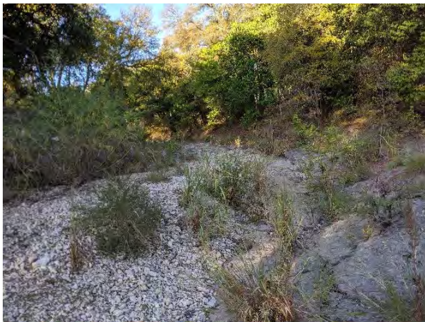
Figure 2-1. U/S of West Gate Blvd near Bayton Loop
