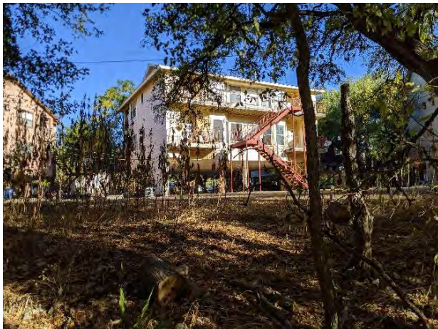
Figure 2-3. Elevated structures on left overbank between Williamson Creek and Sunset Valley Tributary
