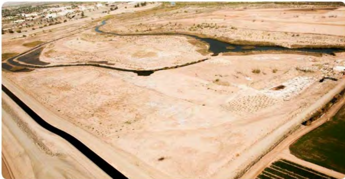
Same site after clearing, grading, and installation of water control structures
