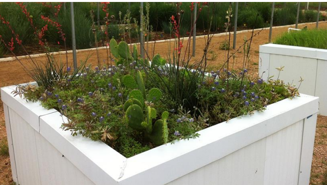
roof trial LBJWFC
