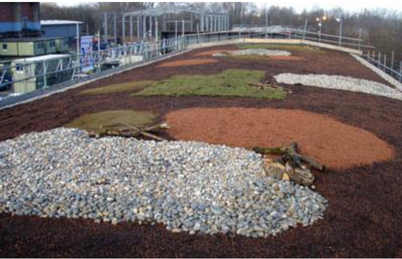
Rubble roof Hackney, UK
