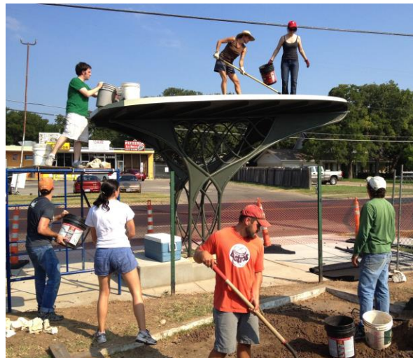
Pecan Springs Bus Shelter
